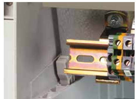
Application of the inner door guarantees IP40 degree of protection when the switchboard door is open.
